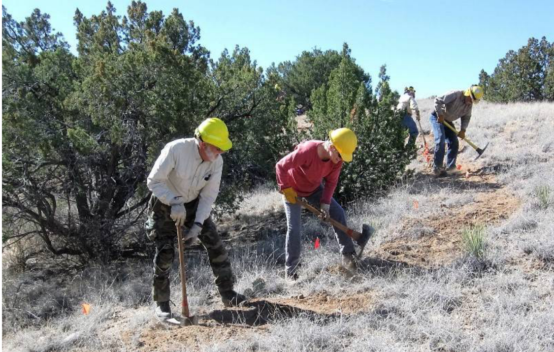
Digging trail tread on Fence Line Trail Photo by Sally Lowder
