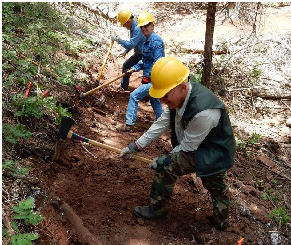
L to R: Jerry Pekarek, Linda McDowell, and Ken Nicholson cutting back slope on Faulty Trail. Photo by Dan Benton
