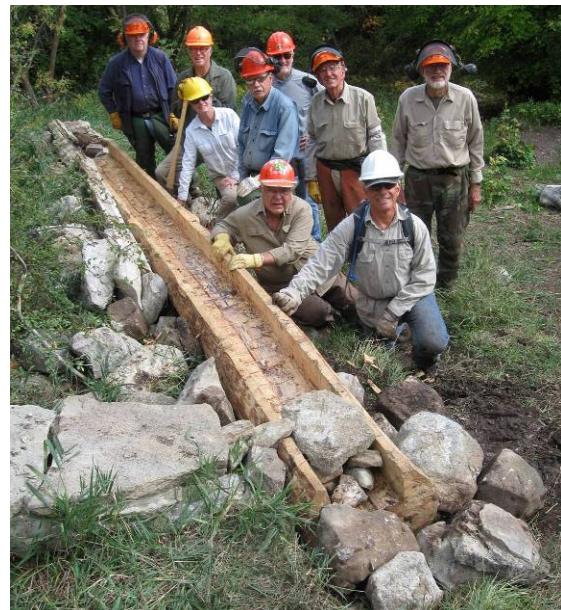
Top – Moving Bird Log onto stone and concrete base in September 2016. Bottom -- Bird Log in final position. A small stream of water from Capulin Spring enters the log under the rocks in the foreground and flows out the far end of the log.
