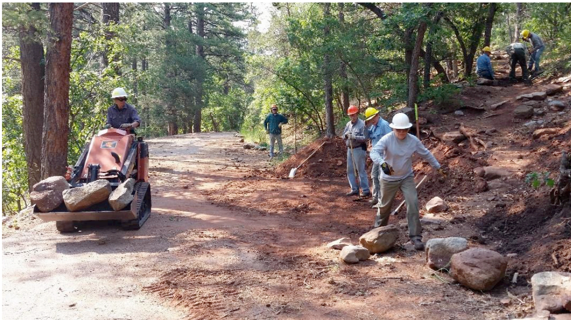
Rebuilding the trail between Doc Long Picnic Area and Sulphur Canyon Picnic Area. Jessica May, USFS, is moving large rocks with the skid steer. Photo by Betsy Galloway
