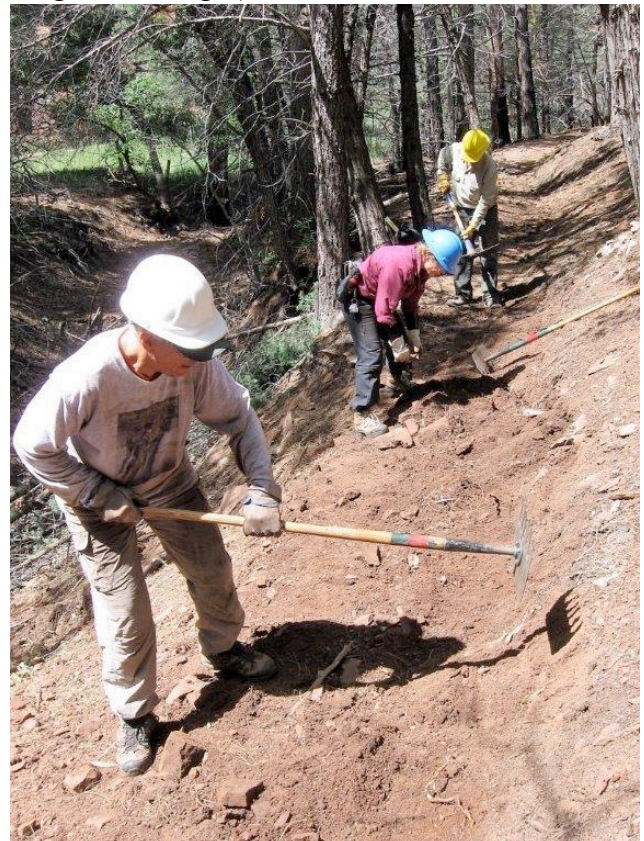
Digging new trail tread on Acequia Trail. L to R: Steve Roholt, Bet Gendron and Jim Levesque. Photo by Sally Lowder
