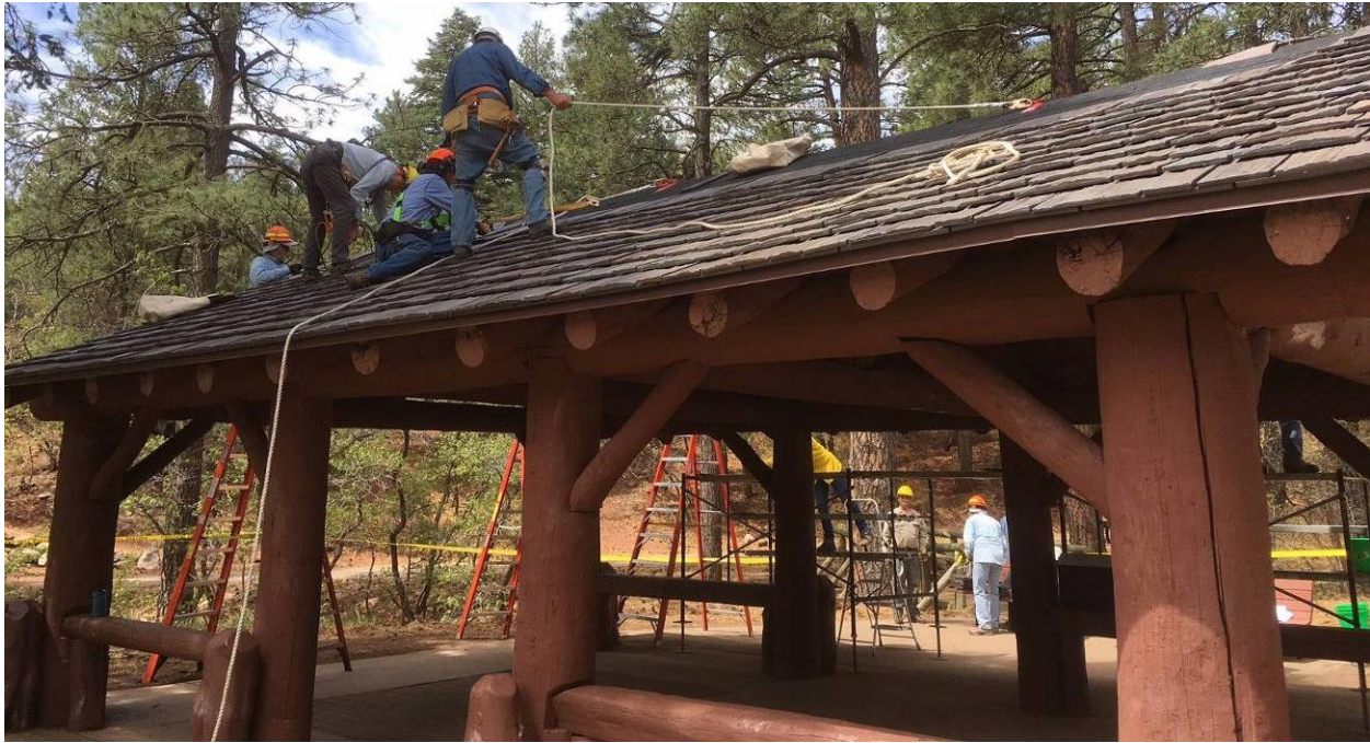
Volunteers putting synthetic cedar shakes on the CCC picnic shelter in Doc Long Picnic Area. Photo by Sam Beard
