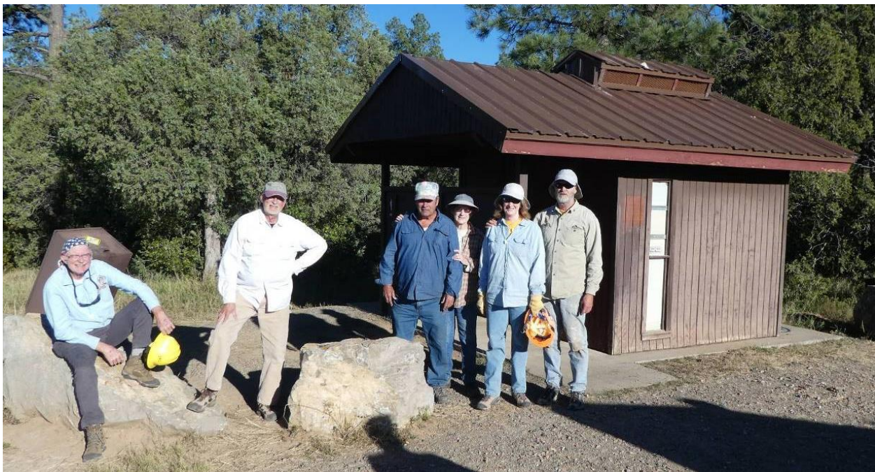
The roofing crew in front of the Pine Flat South Restroom with the new metal roof. L to R: Eric Russell, Dan Benton, Russ and Ellie Parker, and Betsy and Bob Galloway. Photo by Sam Beard
