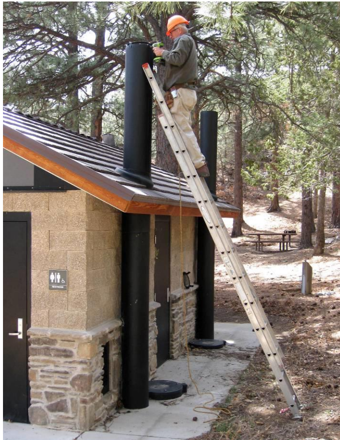
Jim Lunn attaching Poo Poo Screen to the top of a large ventilation tube in Las Huertas Picnic Area. Photo by Carl Smith
