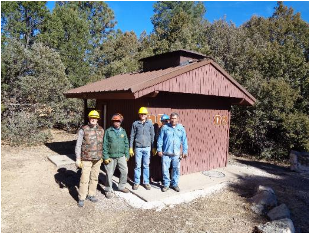
A steel roof was installed on a restroom in Oak Flat Group Picnic Area. L to R: Dan Benton, Jim Levesque, Sim Cook, Ellie Parker, and Russ Parker
