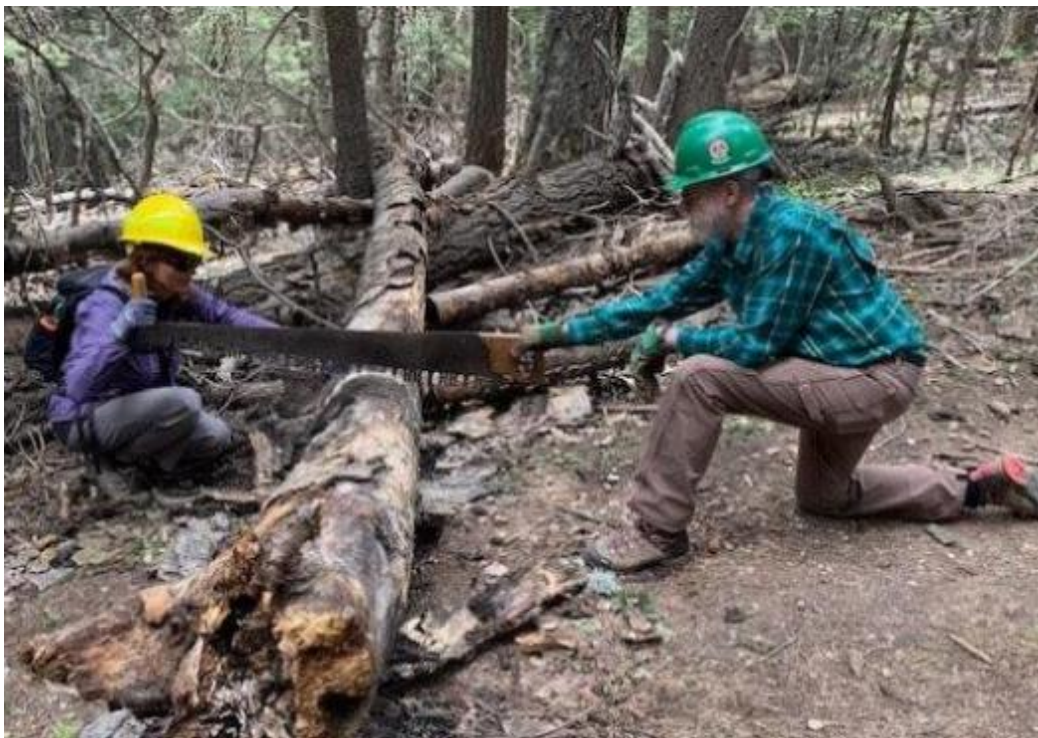
Silke Bletzer and Cleve Sharp using a crosscut saw to remove a log from a trail.
