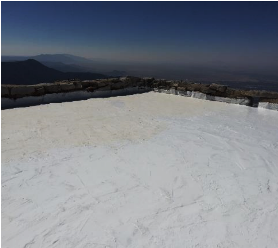
L to R: Sandra Coombs, Joelle Hertel, and Mike Madden are applying a silicone coating on the roof of Kiwanis Cabin.
