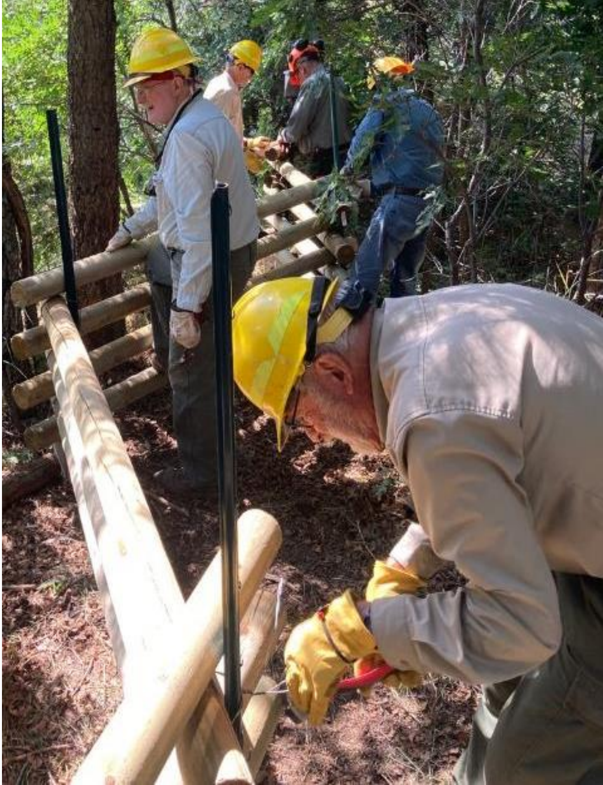
Sam Beard is twisting wire to secure a pole to the steel fence post at the segment of fence being built at Tree Spring Trailhead. L to R: Eric Russell, Sam, Sim Cook, Jerry Carroll, and Jerry Pekarek.
