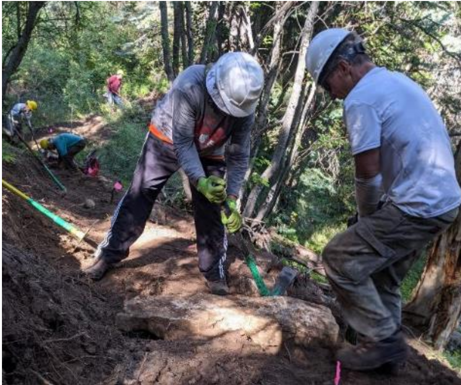
Volunteers are using pick mattocks to remove a rock from a new trail. L to R: Rich Miller and Jeff Huser. Background: Mike Madden, Eric Russell, and Jim Houle.
