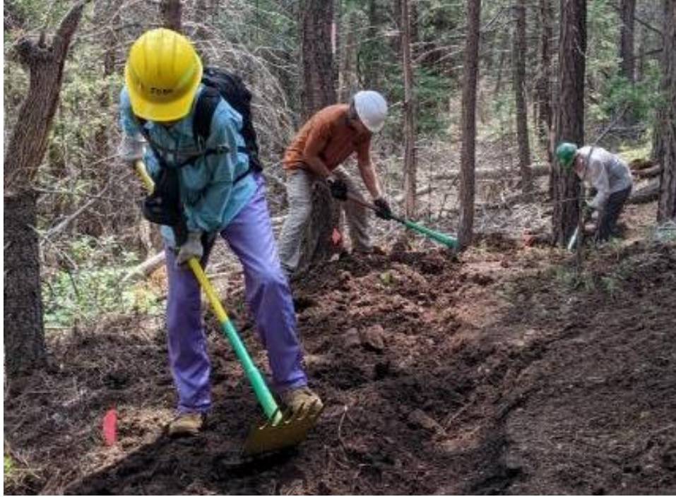
Volunteers using a McCleod and pick mattock to dig a trail tread on a new trail. L to R: Rav Nicholson, Jeff Huser, and Cleve Sharp.
