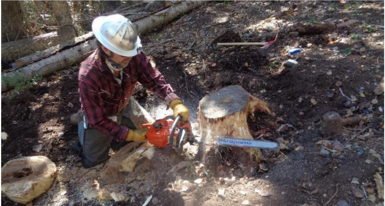
Michael Arndt low cutting a stump on a Sandia Nordic Ski Club trail so that grooming equipment will not hit the stump.
