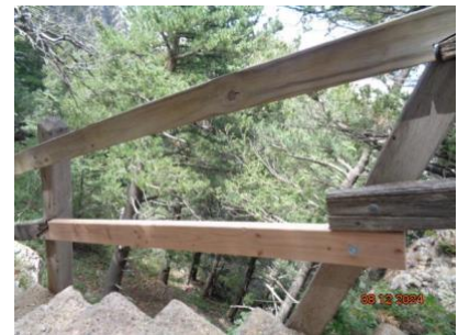
New railing on Crest Spur Trail
