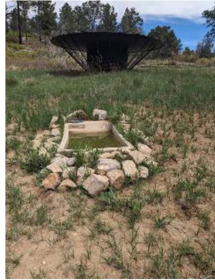
Typical wildlife water installation with rainwater collection and storage in the background
