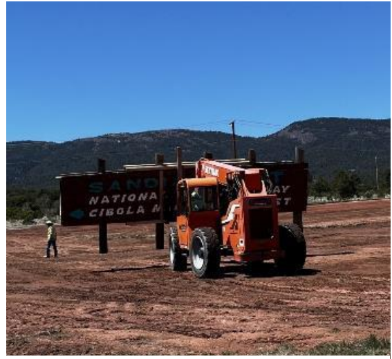
The historic Crest Highway sign being moved to the south-west side of the construction site
