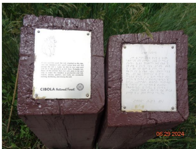
Cienega Nature Trail interpretive signs that have been restored with epoxy paste and paint
