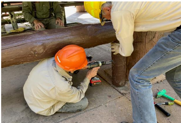
Installing a short post on Doc Long Picnic Area shelter, Don Carnicom and Sim Cook
