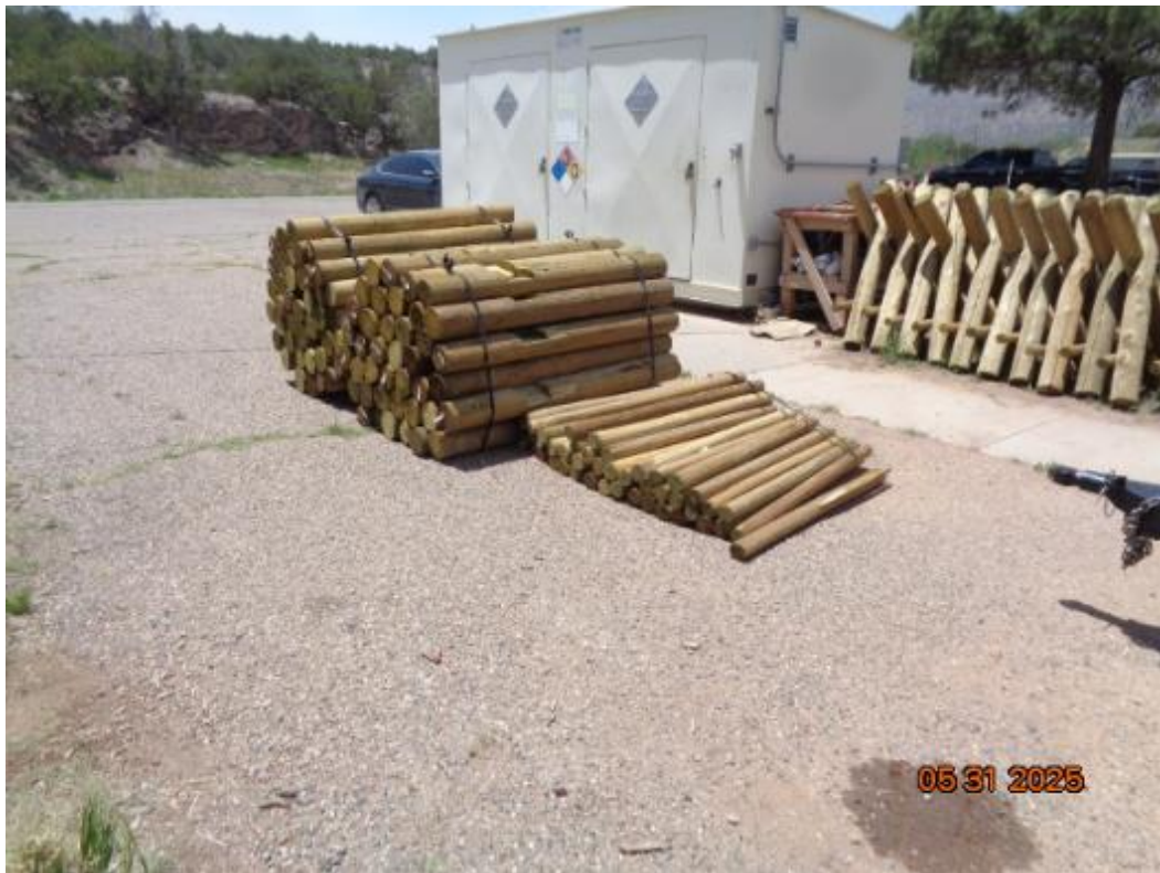
Piles of notched pressure-treated posts, 4-foot braces, and assembled bucks at the hazmat building.
