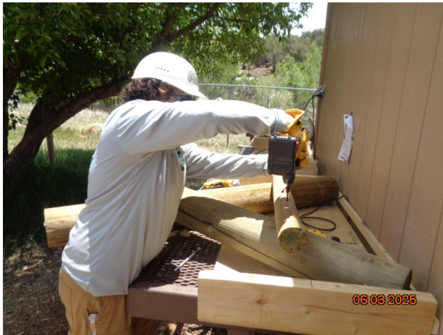
This photo taken on June 3 shows one of the TTYL/YCC crew members making a buck using the jig shown above. The two notched and crossed posts are placed in the jig in the correct position, and a 3-inch by 4-foot brace is placed on the buck legs at a location marked on the jig 2x6 sidewall. An 8-inch or 9-inch 3/8-inch carriage bolt is inserted through a hole in the crossed legs, and a washer and nut are screwed on the bottom of the buck. In this photo, the crew member is using a battery-powered driver to place a 6-inch timber screw through the brace into a leg.
