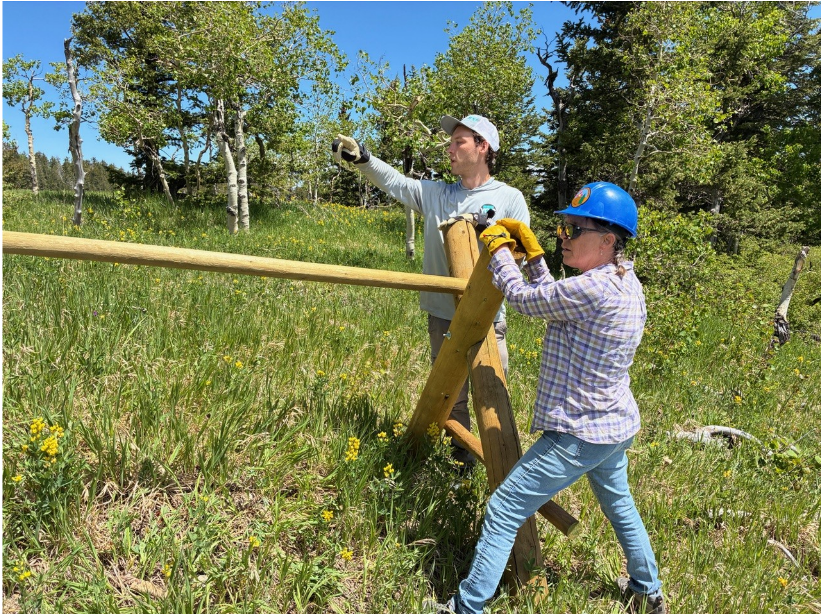
Aidan Stewart and Laura Leon hold a buck for a new section of the fence.
